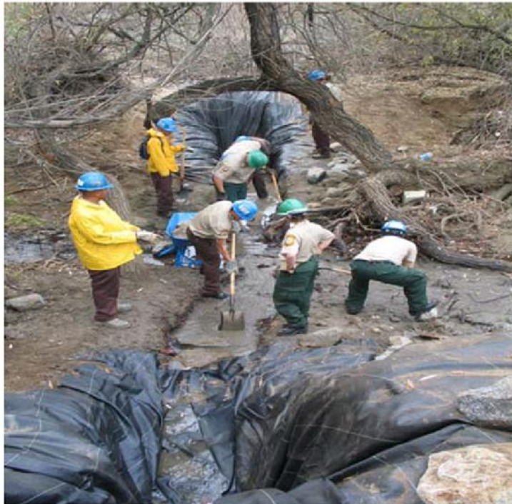
Site of grade stabilizer before installation of keyway. Over 10,000 pounds of rock were placed by hand by crews from the California Conservation Corps to complete the project. Work on the stabilizer began in winter of 2005.
