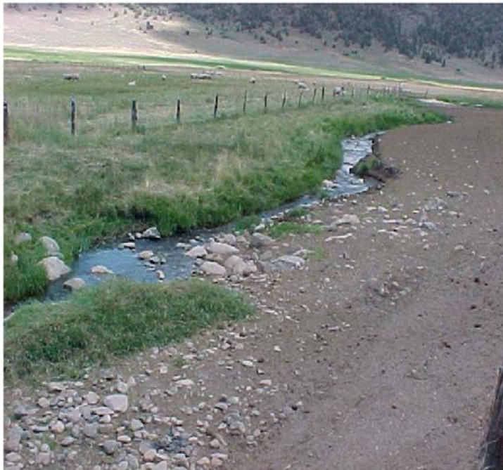
Exclusion Fencing Installed at the Project Site
