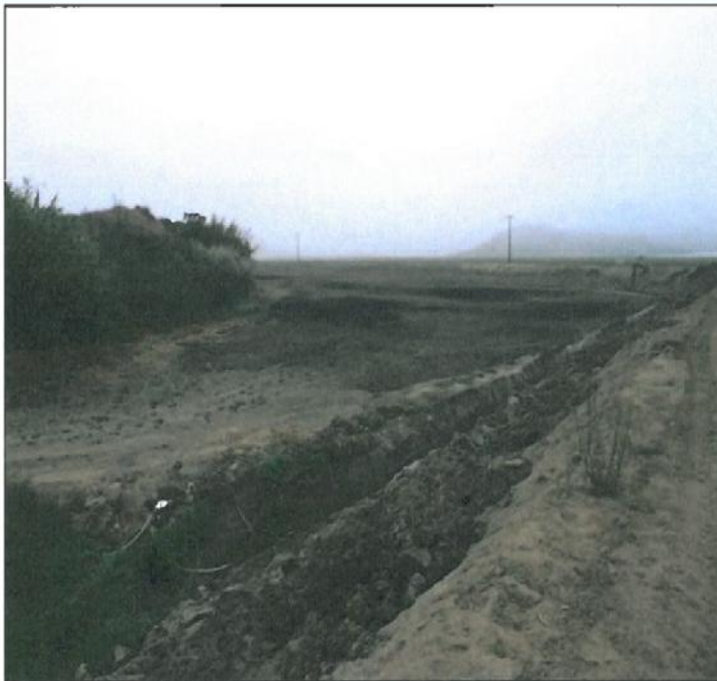
Sediment Basin captures rain runoff and allows sediment to drop out of the water. Capturing sediment also reduced legacy pesticides.
